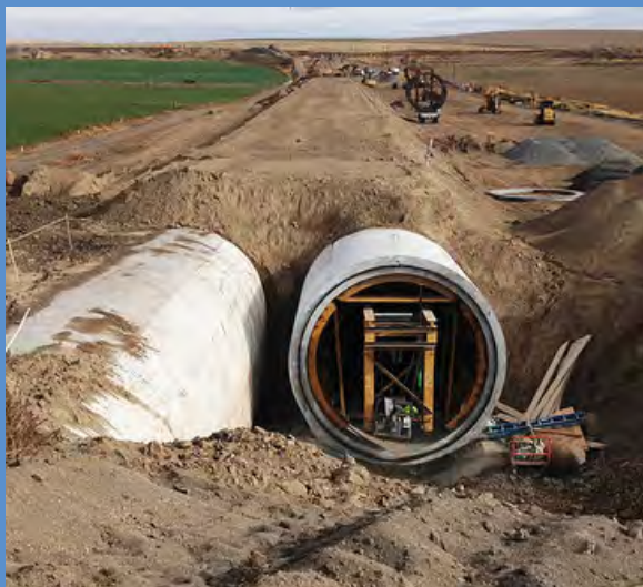
Lind Siphon Completion
